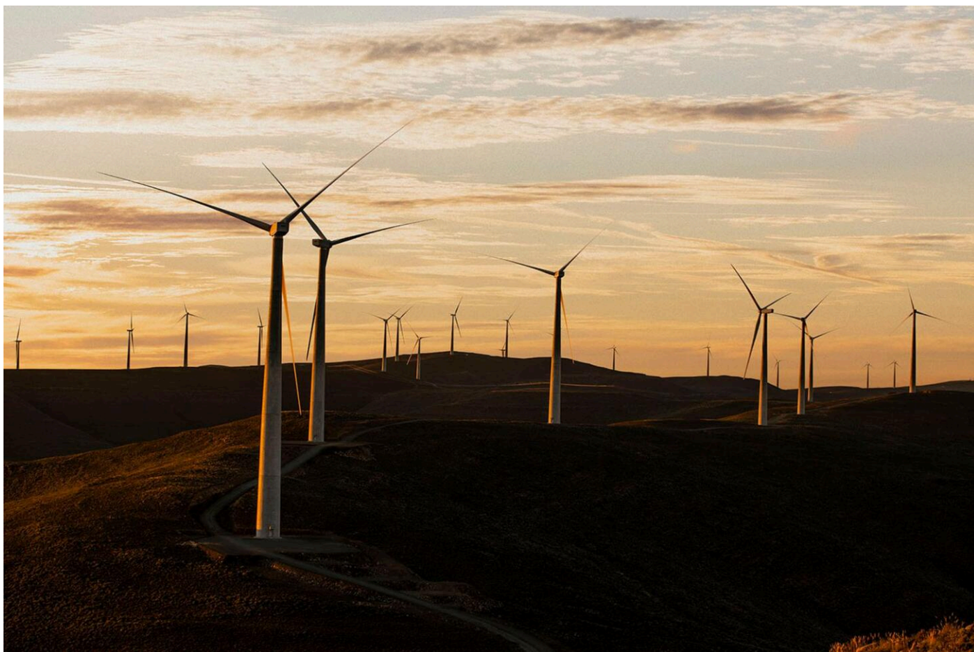
Roggeveld Wind Farm. Picture File
